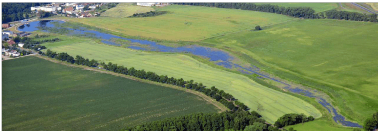
Fig. 2. Przebędowo reservoir – view from the northern side (source: Sojka et al., 2017)
