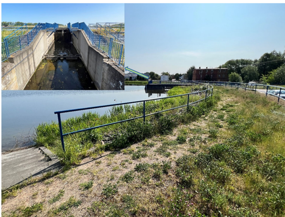
Fig. 3. Earthen head dam with overflow structure on Przebędowo reservoir
