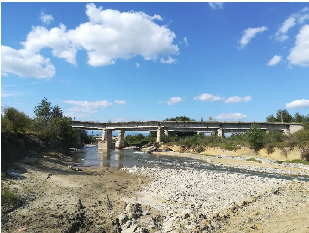
Fig. 8. Railway bridge, Albeni. Photo taken in 2019
