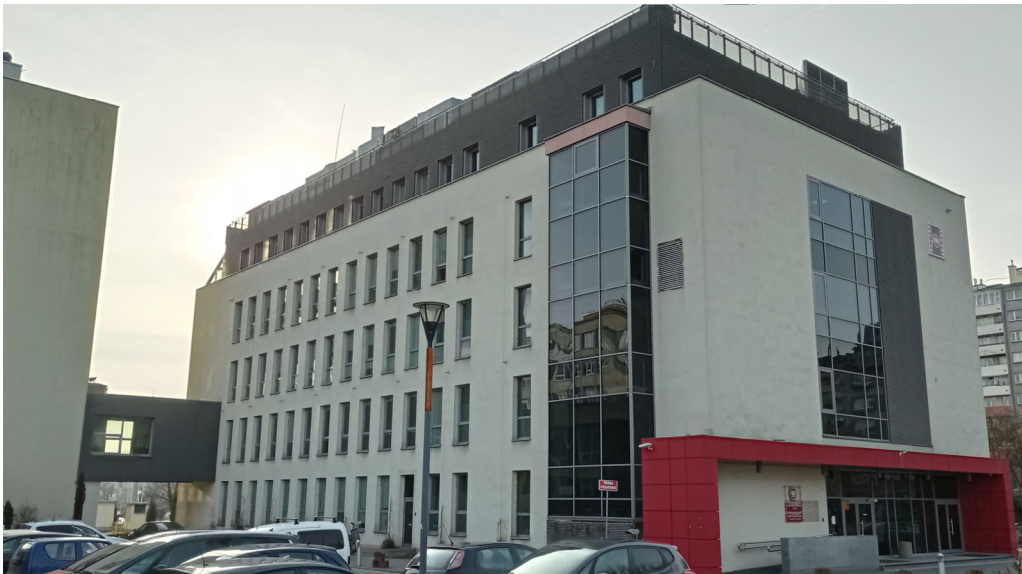
Fig. 1. Intelligent building "Energis" of Kielce University of Technology
