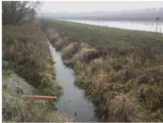
Fot. 1. Urzędówka River – reciver of wastewater from the hybrid constructed wetland wastewater treatment plant in Skorczyce (fot. M. Gizińska)
